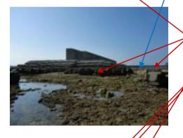
10 t blocks are easily broken down by wave
